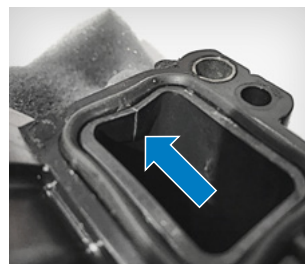
Fig. 2: Breakage (damage pattern)
